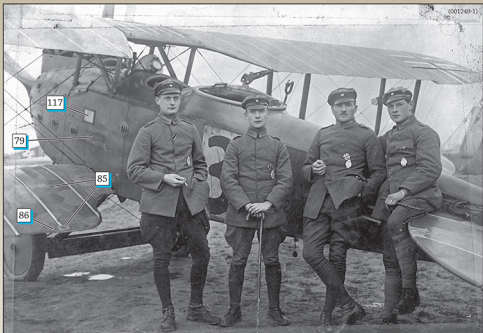
This unidentified LVG C.VI "3" was reportedly photographed on the day the Armistice came into effect. Note the 4 colour lozenge fabric, angle of incidence stencils 86 and ZaK inspection windows 85 .
