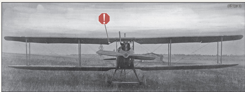
Front view of LVG C.VI 7631/18 showing battle damage to the inner starboard top wing. Note the washout of the ailerons.
